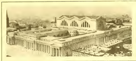
General view of the Pennsylvania Terminal in New York City.
